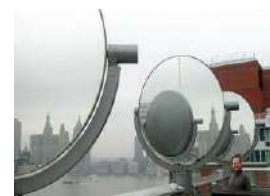
Figure6 A heliostat used in a sustainable building to collect and redirect daylight.
