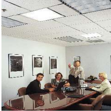
Figure15 The building has modular daylight system in addition to a backup electric modular system. The daylight system saves 23% of energy used in lighting.
