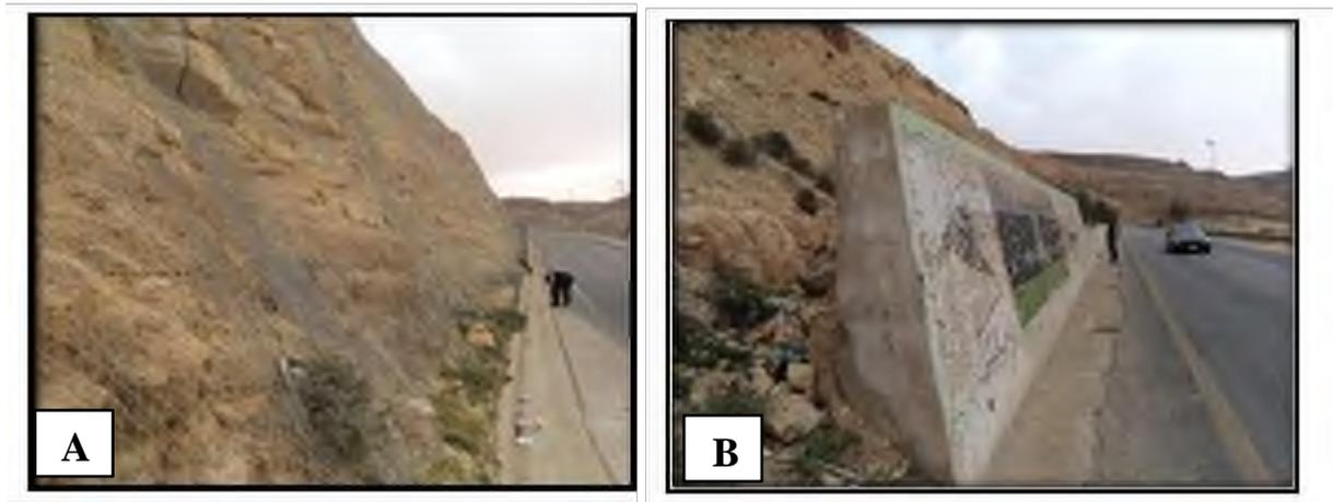
**Photograph 3 (A - B).** Showing the use of metal nets fences and concrete walls to prevent the rockfalls of Ain Tobi Member.
